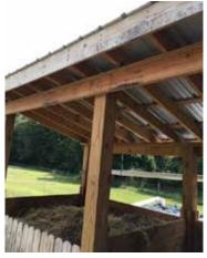
Composting bins don't require a roof but having one helps maintain the proper temperature of the compost by keeping the material warmer in the winter. It also allows the property owner to control the amount of moisture.
