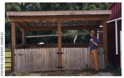
Front view of a two-bin composting system. This system is designed to accommodate the manure from three full-sized horses.
